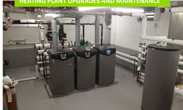
HEATING PLANT UPGRADES AND MAINTENANCE
