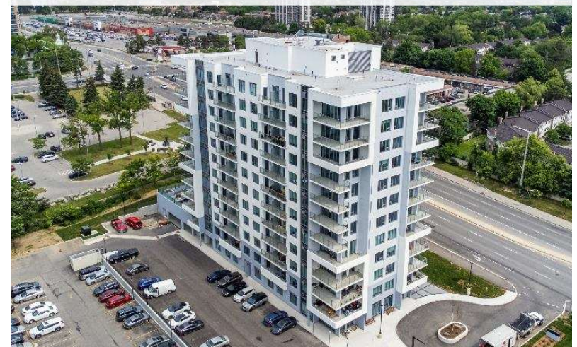
The Kay – Geothermal Heating & Cooling
